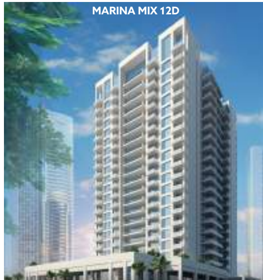
Owner: Assets Real Estate Development | Location: Marina Dist - Doha, Qatar | Floors: 3B+G+21
